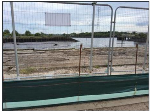
Photograph F-4 - BH107 with in-situ silt fence associated with existing construction zone
